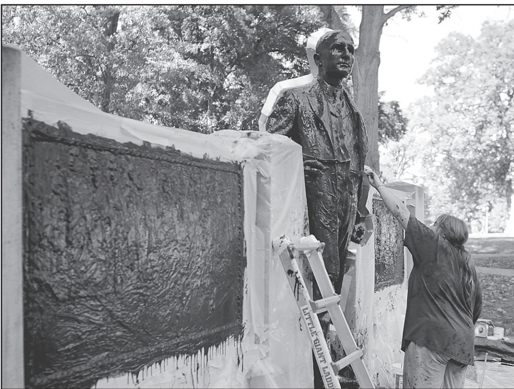
Doreen Bledsoe prepares the rubber-coated C. B. Aycock statue to accept its upcoming layers of supporting plaster.
