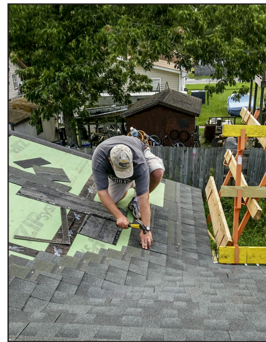
Crews were roofing the day Masons volunteered.
