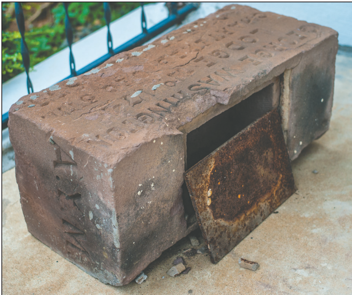
After a report from a neighbor, Columbus Lodge members found the long undisturbed cornerstone of George Washington Lodge cracked open on their porch.
