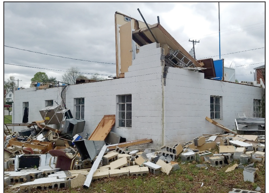
Damage caused by a tornado was extensive in Greensboro, destroying a Prince Hall lodge building. Debris was scattered around the property, including lodge furnishings and art work.
