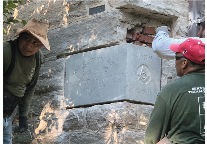
Workers carefully extract the cornerstone from the former temple.
